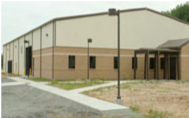
Coal Mine Training Center at Rend Lake College. Image Credit (both images): RLC
