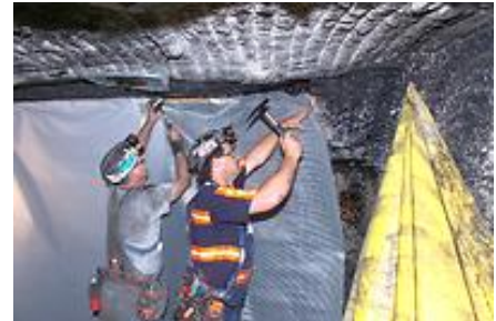
Installing a ventilation curtain.
